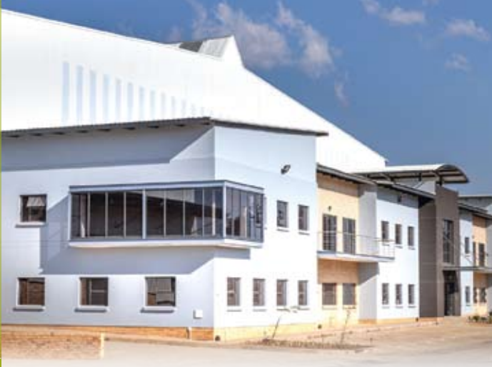
Mostyn Park Randburg – Renico's flagship warehouse to Tiger Brand's specification
